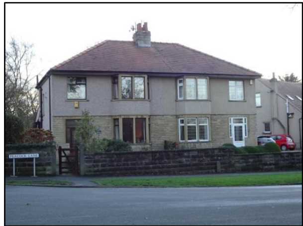
Photo 14. Semi-detached houses on Peacock Lane
